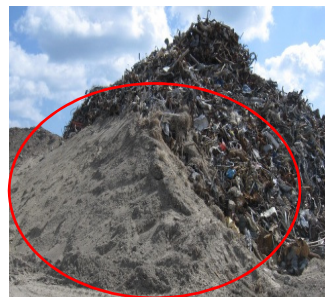
Fig. 5 Slope covers to restrict oxygen inflow
