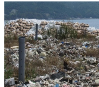
Fig. 6 Pipes for the release of heat and gas monitoring
